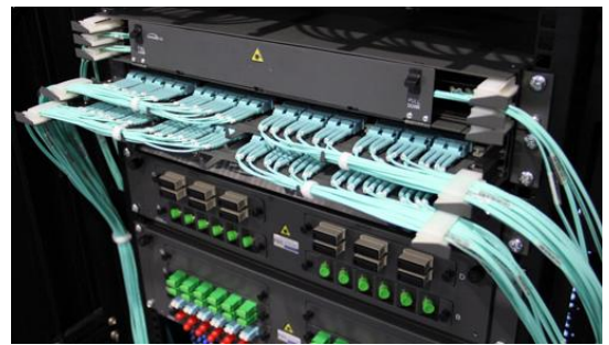
Individual sliding trays for each row of cassettes allow for simple patching, cassette insertion and removal and unparalleled finger access
