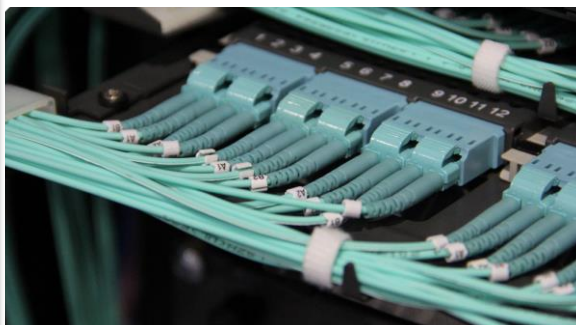
Clear port labelling, excellent fibre routing, excellent finger access and simple patch lead retention without the need for specialised patch leads
